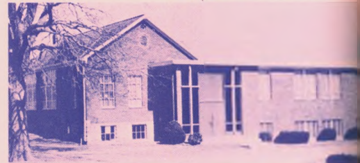
Present Liberty church building, purchased from another denomination.
